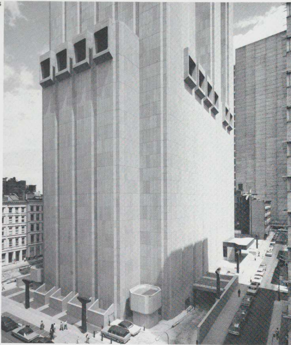
36. John Carl Warnecke & Associates. New York Telephone Company Equipment Building, New York, N.Y. 1966-72
