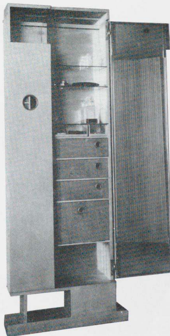
Dressing cupboard, of aluminium and cork, seen at the right of the illustration on the preceding page. It faced into the master bedroom lavatory and when opened revealed drawers and shelves for toiletries and, on the inside of its door, a full-length mirror.
