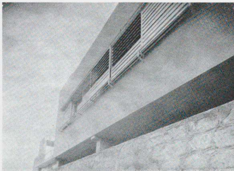
Throughout the house sliding windows and shutters set in tracks are used for privacy and protection from the glare of the sun.
