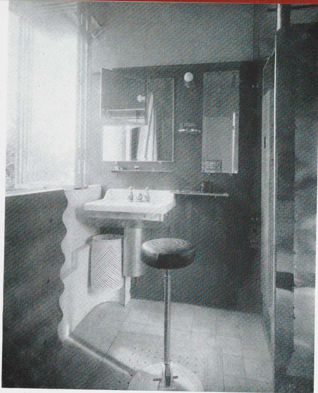
Lavatory at the end of the master bedroom. One section of the mirror above the basin turns to adjust the reflected image. The ingenious design for windows, which slide to one side on tracks, was patented by Jean Badovici in 1929.
