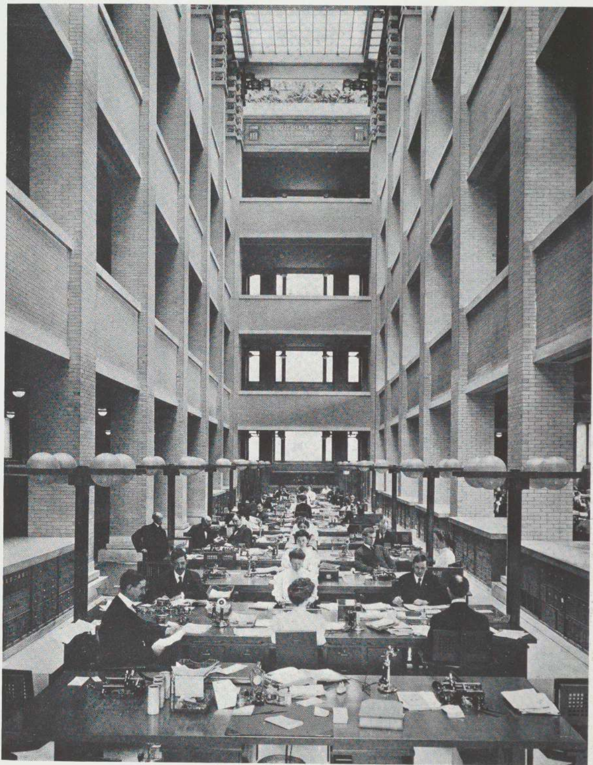
FRANK LLOYD WRIGHT: ADMINISTRATION BUILDING, LARKIN SOAP FACTORY BUFFALO, N. Y. 1904-1905—Interior
