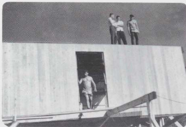
6. Stamos House under construction, with Tony Smith (top left) and crew, 1951
