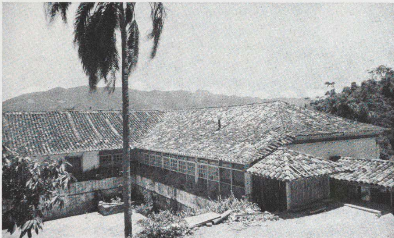
Old house near Rio. A continuous band of glass and lattice opens on the greenery of a great cantilevered window box
