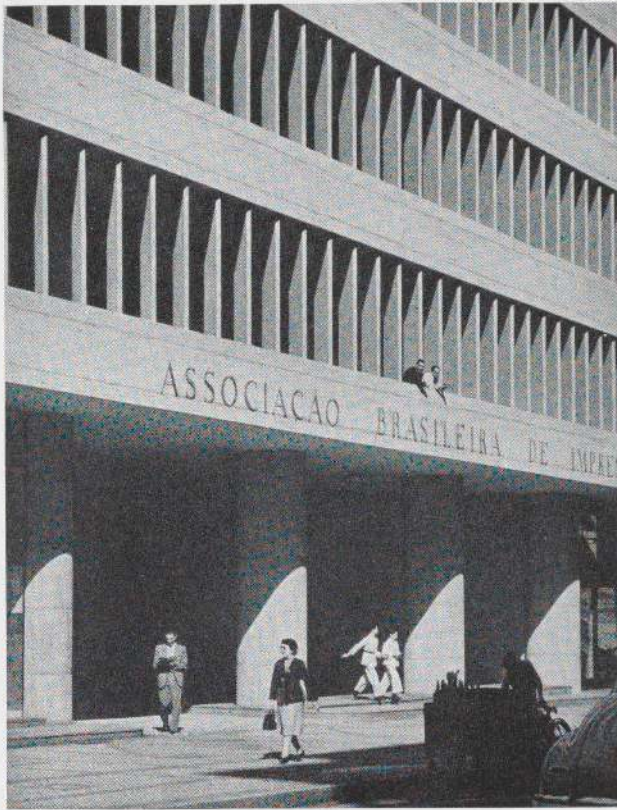
The A. B. I. has fixed concrete blinds
