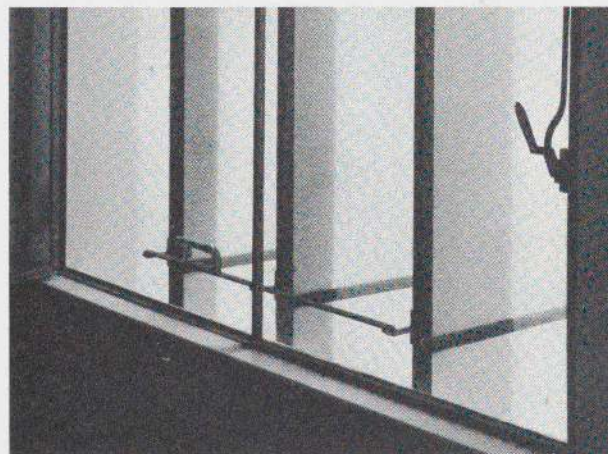
Simple mechanism which adjusts the blinds of the Day Nursery
