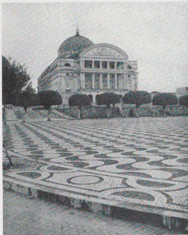
Opera house in Manáos
