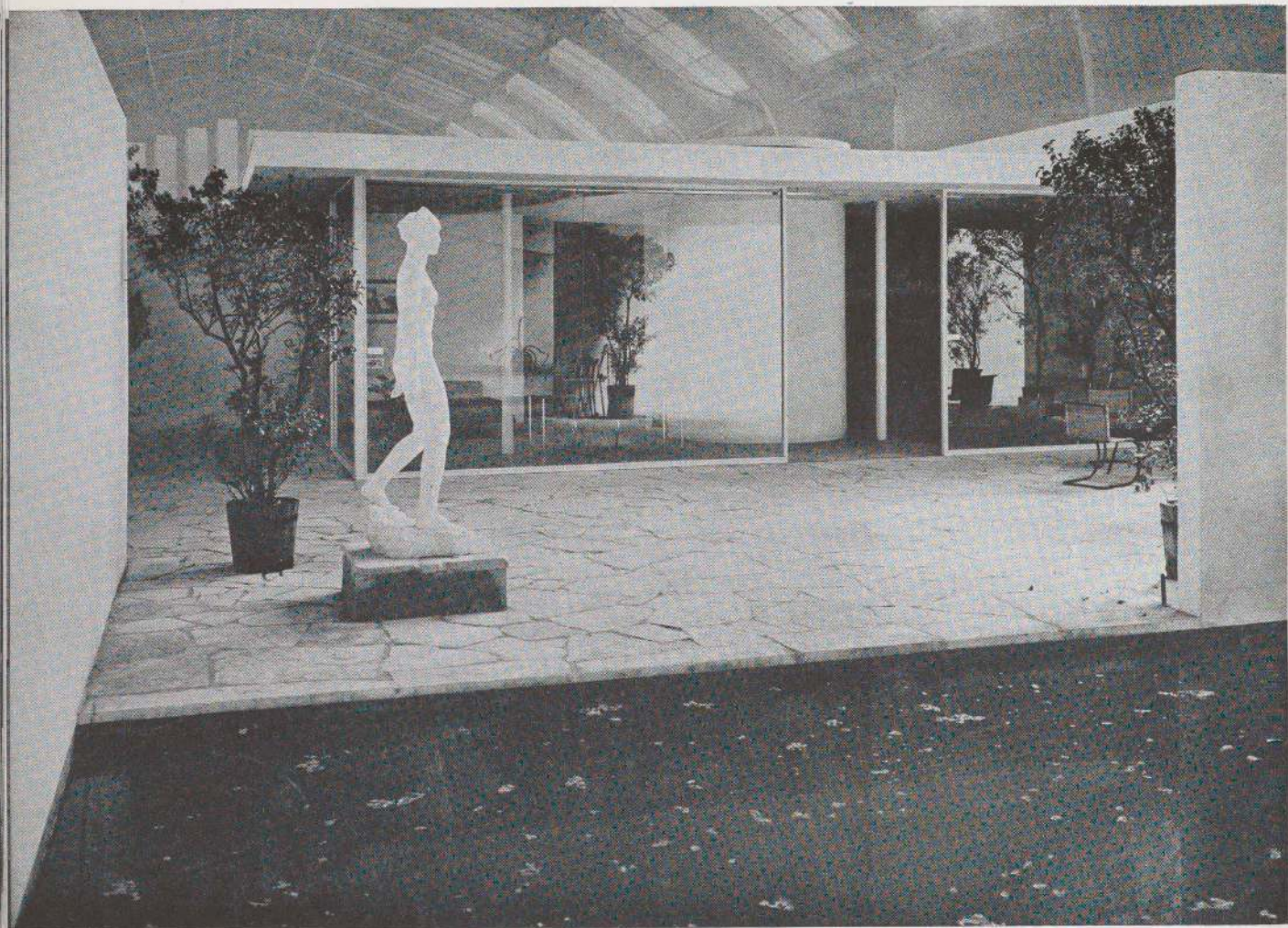
House, Berlin Building Exposition. Enclosed garden
