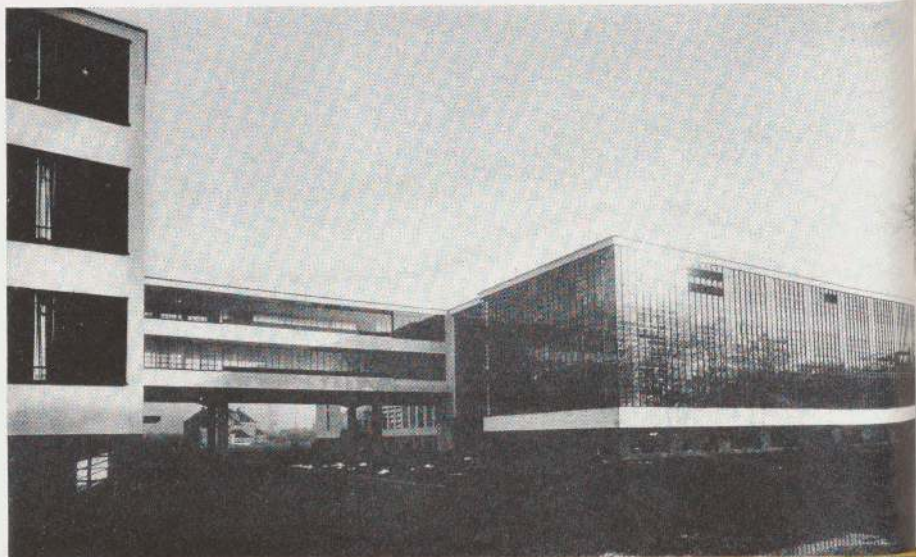
Walter Gropius: Dessau Bauhaus. View from south- west. 1925-1926
